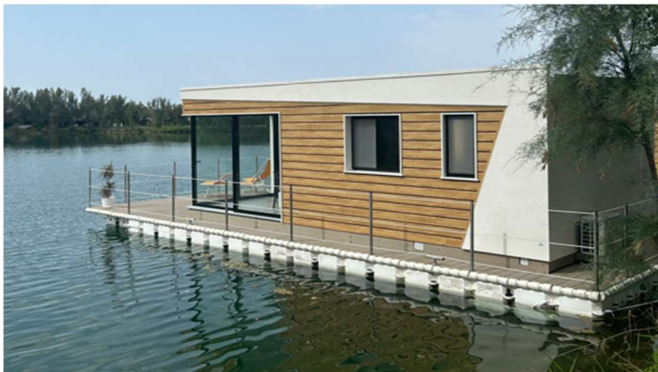
Floating Construction - Italy
